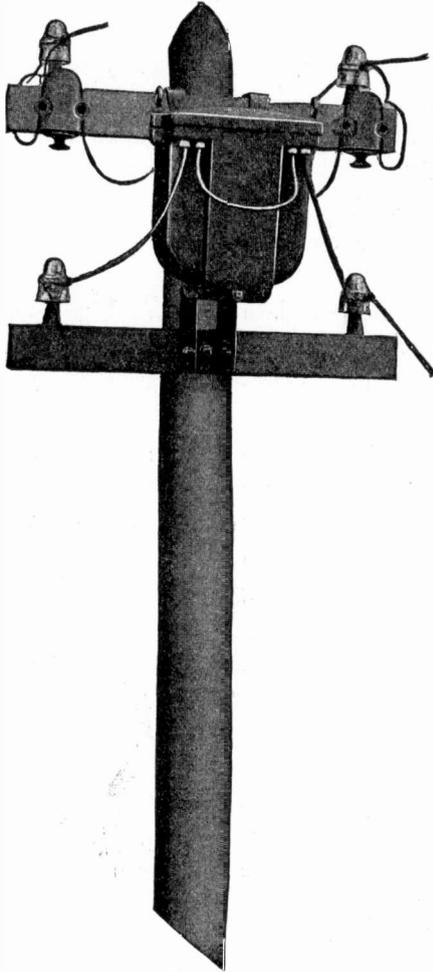
Fig. 274. Method of Connecting Wires to Primary Fuse Block on Poles Before Current Passes to Transformer
