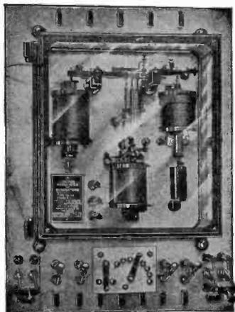
Fig. 86. Front View of Generator Voltage Regulator
