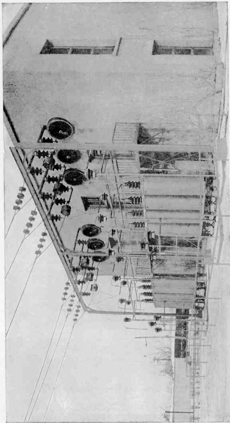
**LIGHTNING ARRESTERS ON INCOMING LINES AT SUBSTATION**
