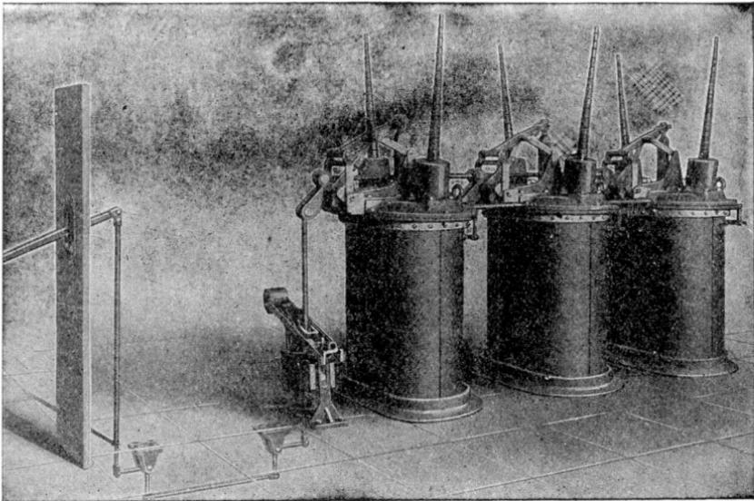
Fig. 385. Westinghouse Three-Pole Oil Circuit Breaker—"Remote Control"
