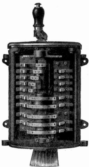
Fig. 337. Westinghouse Controller for Induction Motors
