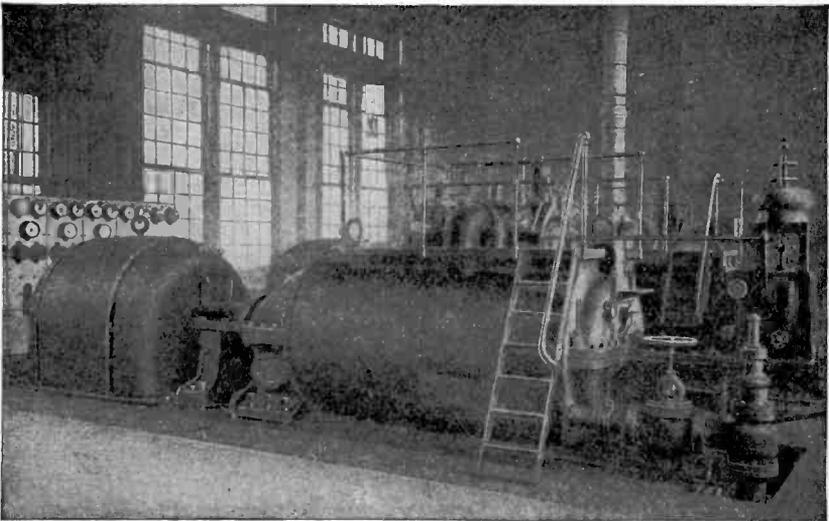
Fig. 150. General View of Westinghouse-Parsons Three-Phase Four-Pole Turbo-Alternator
