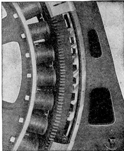
Fig. 133. Portion of General Electric Alternator Showing Method of Dovetailing Core Laminations
