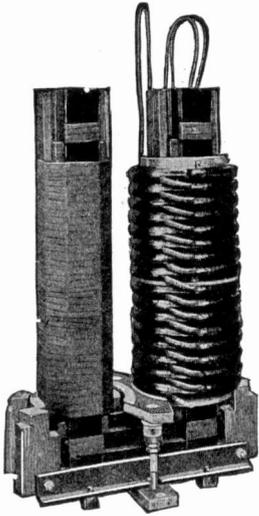
Fig. 234. General Electric Core-Type Transformer Partly Assembled
