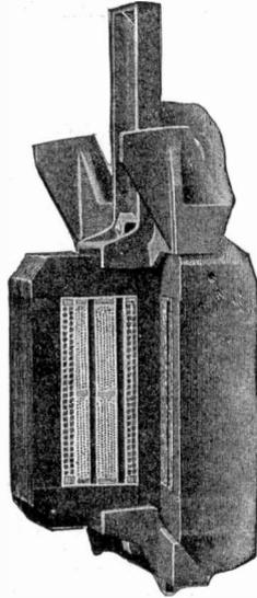
Fig. 249. Part Section through Westinghouse Transformer
