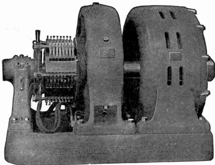
Fig. 316. General Electric Motor-Generator Set—Induction Motor Driving Compound-Wound D. C. Generator
