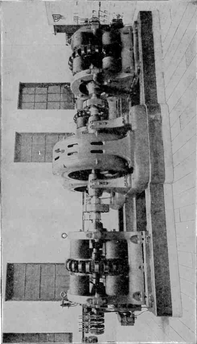
Fig. 317. Two Sets of Brush Arc Dynamos Direct Connected to Induction Motors
