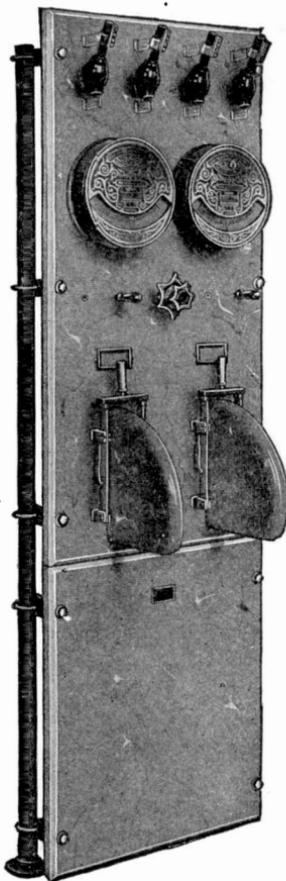
Fig. 366. Standard Switchboard for Single-Phase Generator and Two Feeder Circuits
