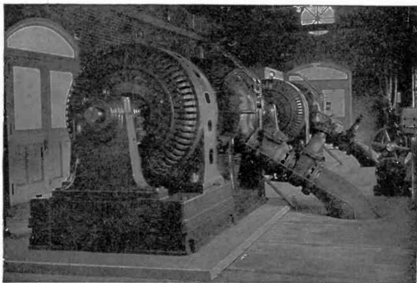
Fig. 346. Westinghouse 500-H.P. Induction Motors Operating Centrifugal Pumps in a Municipal Pumping Plant
