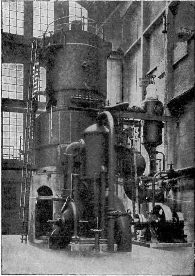
Fig. 154. Curtis Vertical-Shaft Turbo-Alternator of 5,000-Kw. Capacity
