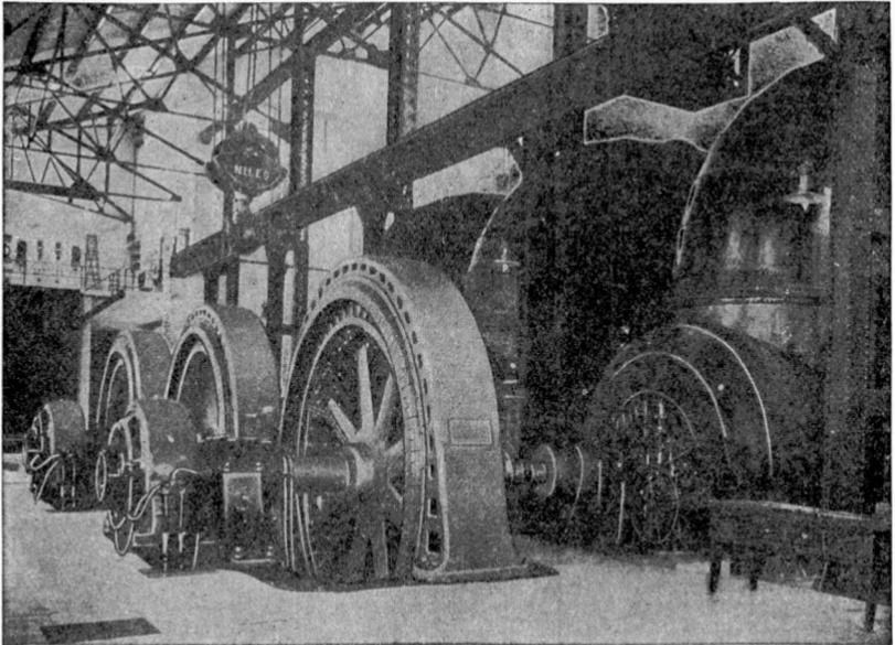
Fig. 146. View of General Electric Water-Wheel-Driven Alternators
