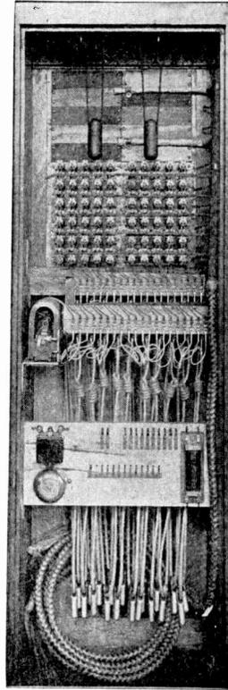
Fig. 143. Upright Magneto Switchboard—Rear View
