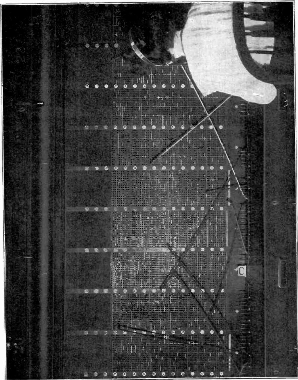
Fig. 220. Section of Trunk Switchboard
