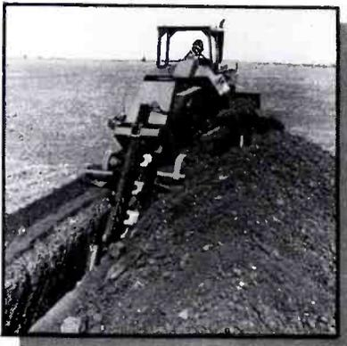
*Ditch Witch: conveyor spoils delivery system*
