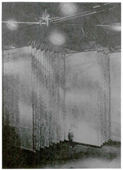
Clifden Station. Main condenser (H.F. Transmitting circuit) was exactly the same at Glace Bay. Photo gives an idea as to size of plates. Beaton Institute
