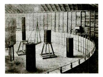
The components of Tesla's large magnifying transmitter inside its protective ring. He was surprised by the heat of the Colorado sunlight. Indeed, it took him so much by surprise that his equipment was damaged because he carelessly left it in the sunshine. A transformer and several barrels of concentrated salt solution were melted and ruined by the heat, and a wooden ball, coated with tinfoil, actually caught fire.
