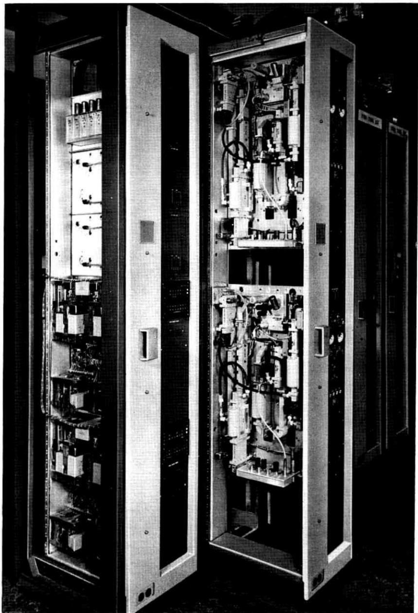
Fig. 8 — Bay arrangement for auxiliary radio channels.
