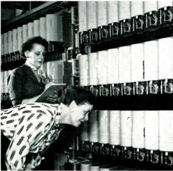
*Fig. 1 — Miss Edna Lazarns, left, and Miss Florence Gorman of the Laboratories record at regular intervals the number of switches engaged with calls. This “switch count” procedure is still widely used to determine usage of dial equipment.*
