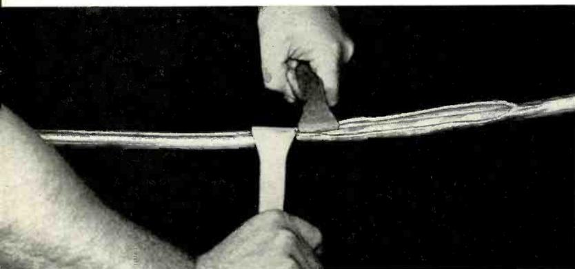
*Tools used to open the sheath wider to permit work on a defective portion of the cable core.*
