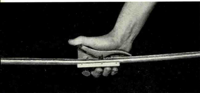
*By means of the cable sheath slitter an incision of the required length is made in the sheath.*
