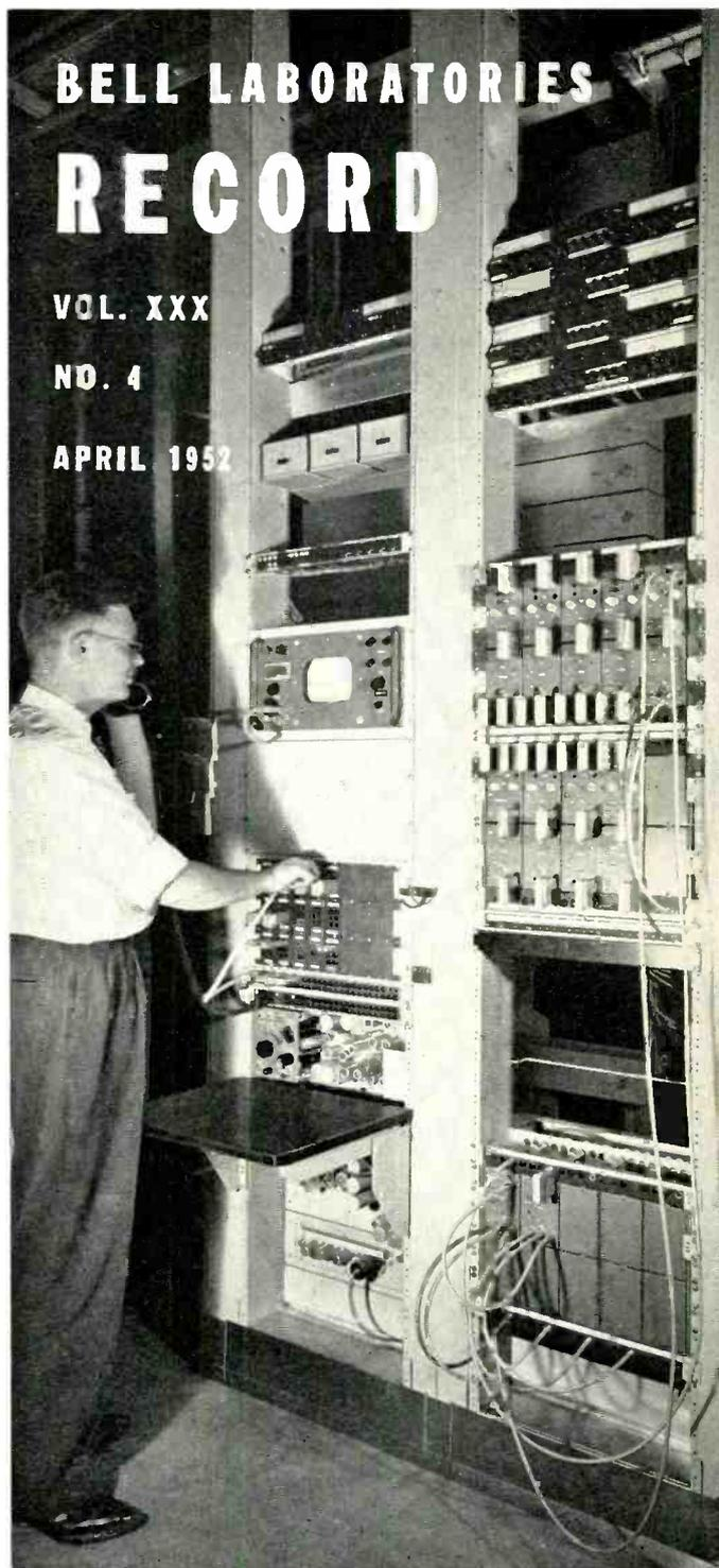
*Monitoring and patching bays. The jack field under the operator's hand provides access to incoming line facilities and to FM terminal circuits.*
