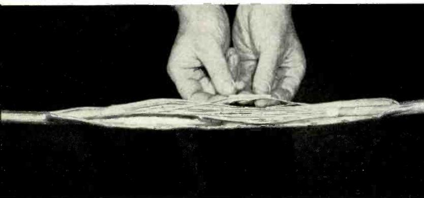
*Insulation is repaired with tape and, at this stage, any wet spots dried and necessary conductor repairs made.*
