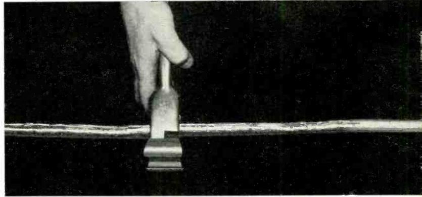
*The cable is sealed against the weather and the repair operation is completed by soldering the opening using an acetylene torch.*
