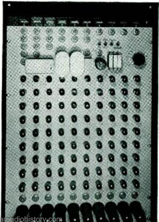
Fig. 1—The analyzer panel with message registers above and the driving tubes below
