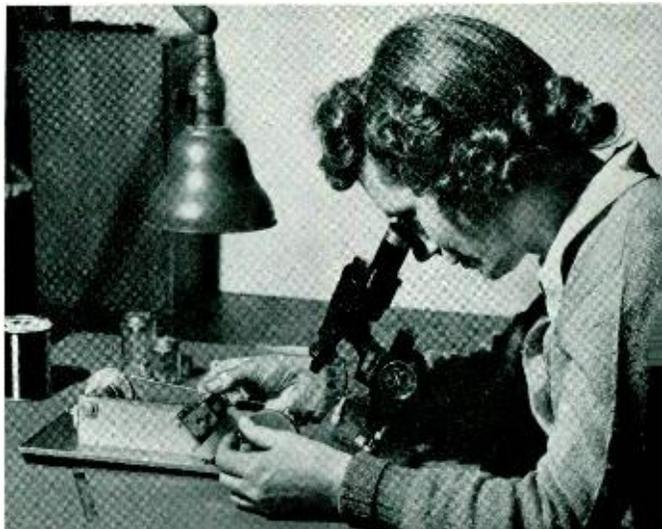
*There are still many mechanical operations too delicate for any but the human touch. Here Carol Ozmac winds wire as fine as a human hair onto the smallest non-linear coil now in production, used as a harmonic generator*
