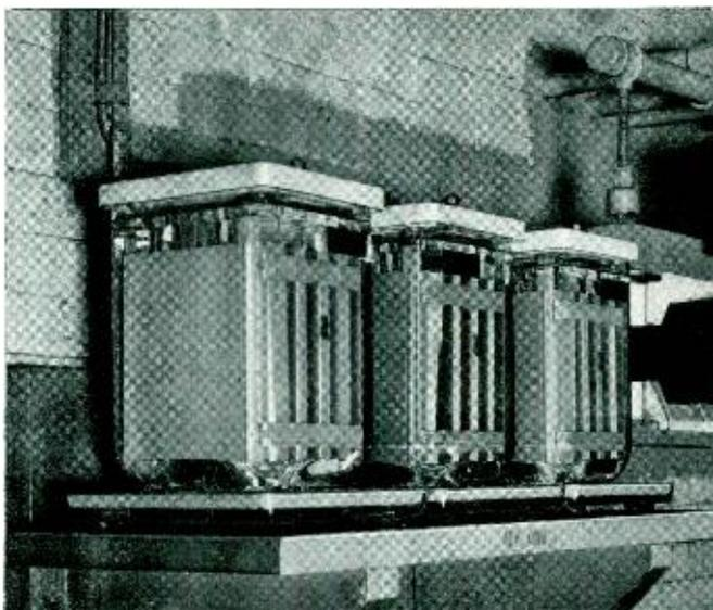
*Electrolytic condensers installed in connection with a 48-volt battery supply in Reading, Pa.*
