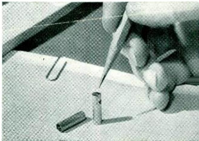
*Contained in a small metal cylinder, the Transistor consists of two extremely fine wires whose points rest on a small square of a semi-conductor*
