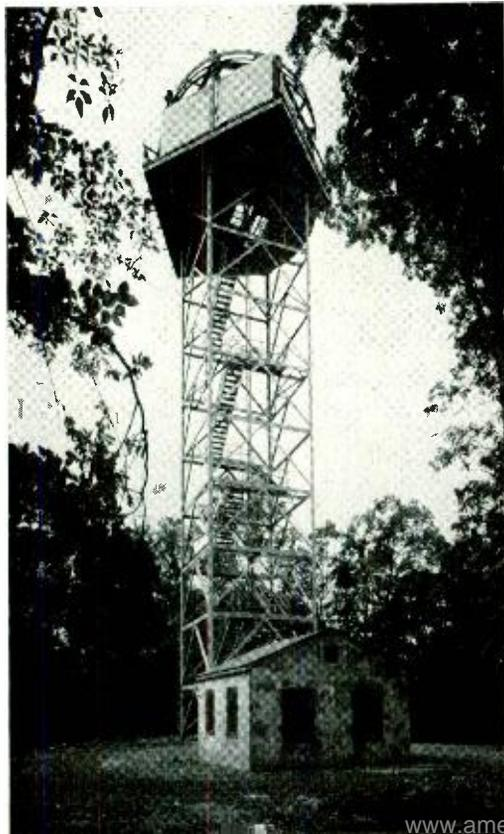
Fig. 1—The 100-foot antenna tower and repeater house at Murray Hill
