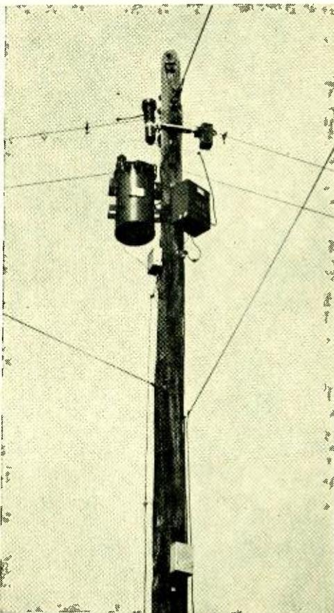
*Subscribers would be connected to the power line through a coupling unit consisting of condensers and a transformer installed on a cylindrical core as shown at the left near the top of the pole beneath the power-line lightning arrestors*
