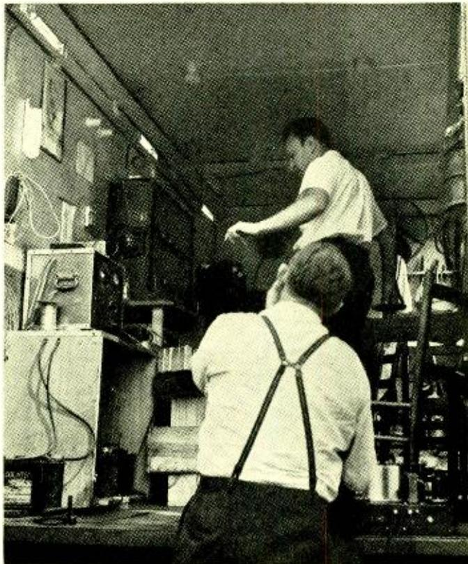
*Interior of Bell Telephone Laboratories' test truck used for transmission measurements on power-line carrier channels*
