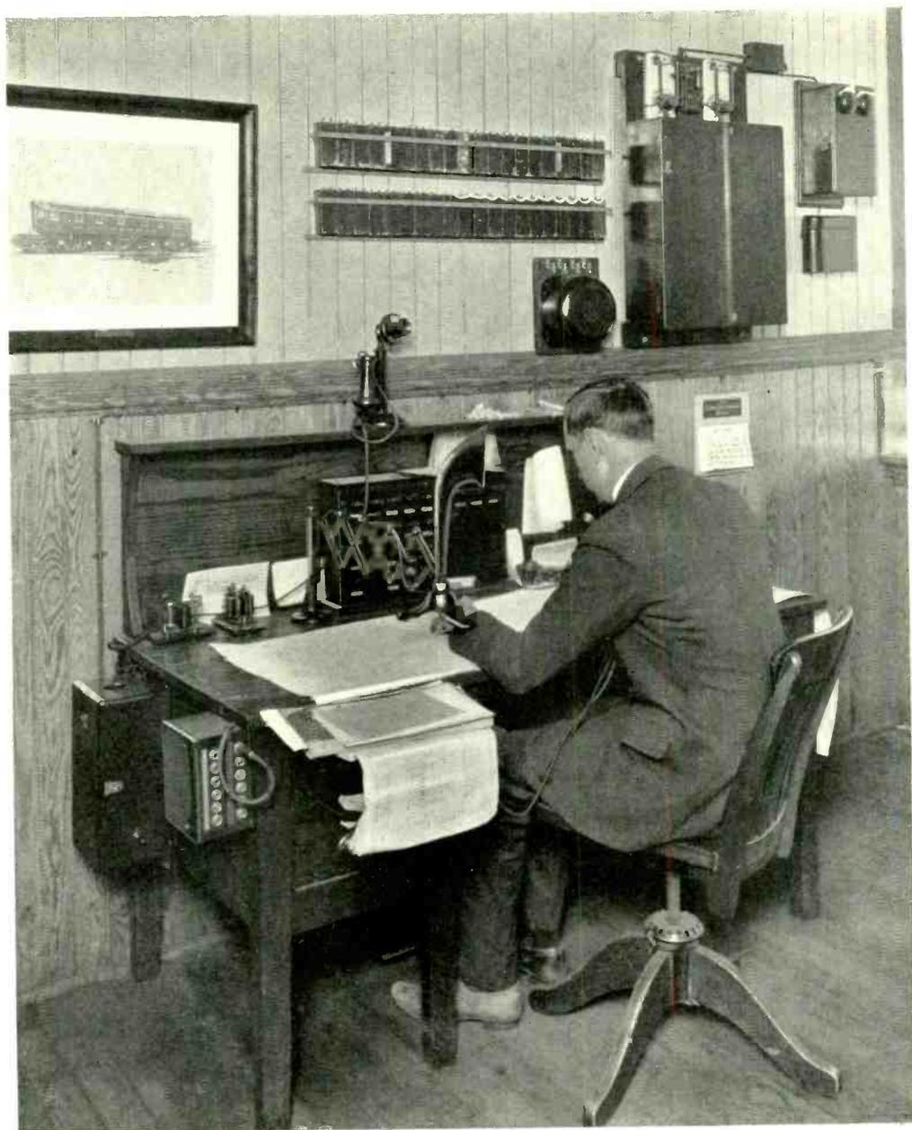
*A typical dispatcher's desk equipped for telephone operation. To the left is a loud speaking receiver; in front of the dispatcher is the bank of rotary keys*
