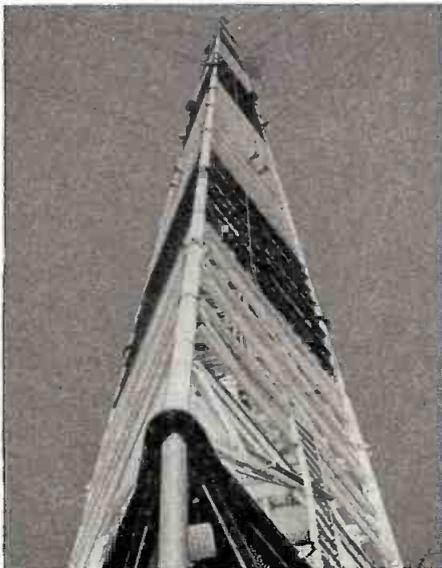
pending FCC approval, another 300 feet of height will bring it to an ultimate 1,499 feet. The tower had to be built with the strength to accommodate this extra weight without the necessity of future structural modifications.
