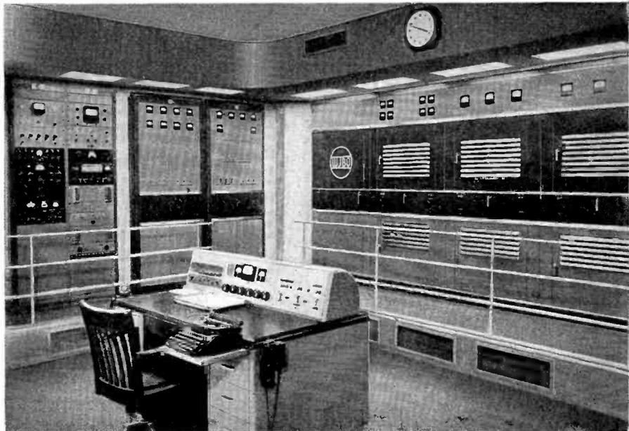
The transmitter room shared by WBRL and WJBO. The 1 kW FM Transmitter is the unit just left of center in this picture. At the far left are racks containing the FM audio input and monitoring units. At the right is the 5 kW AM transmitter. Not shown in this picture are the AM audio and monitoring racks and AM phasing units. All of the equipment in this picture is of RCA manufacture.
