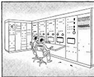
**MASTER CONTROL BOARD.** The Master Control Board is the heart of the television station. Engineers manipulate shading and other controls to add technical refinements with electronic artistry to all programs.
