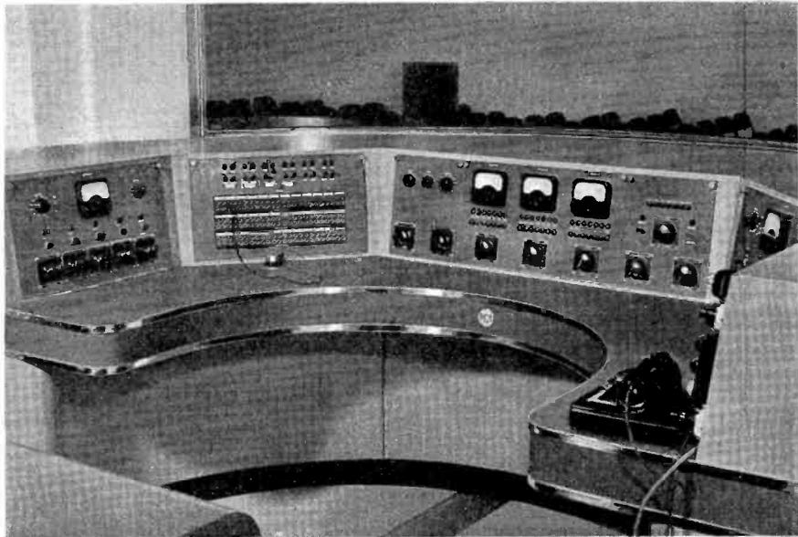
The specially built RCA control console in the master control room shared by WBRL and WJBO. Individual panels control the output from three studios. Network lines and remotes are controlled from a fourth panel. The push-button selector system in the center panel allows any program to be fed to each of the three output lines (one AM, one FM, one spare or network).
