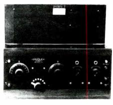
CROSLEY'S EARLY VERSION MODEL VI (SIX) WAS A 2-TUBE TRF RECEIVER USING TWO WOODEN "BOOK" CONDENSERS. IN REALITY, IT IS THE RETA AND HARKO SR. COMBINATION IN ONE CABINET. IT SOLD FOR \$28 WITHOUT TUBES, BATTERIES OR PHONES IN LATE 1922. THIS PARTICULAR MODEL VI IS IN THE "SPECIAL" CABINET WITH ROOM FOR DRY CELL BATTERIES.
