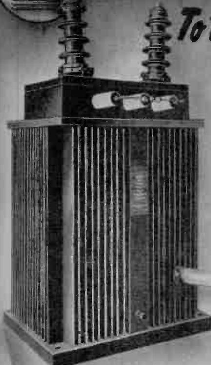
Typical of the large broadcast equipment manufactured by UTC is the filter choke illustrated on the left, designed for a 100 KW broadcast station and weighing about 3 1/2 tons. This unit is 100,000 times the size of the UTC OUNCER.
