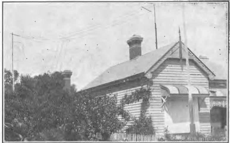
Above photograph shows the aerials of the Wireless Set of Mr. J. Ellis, of Bendigo, Victoria. They are of the T pattern, 50 feet high, with three stranded 7/18 wires. (See opposite page.)
