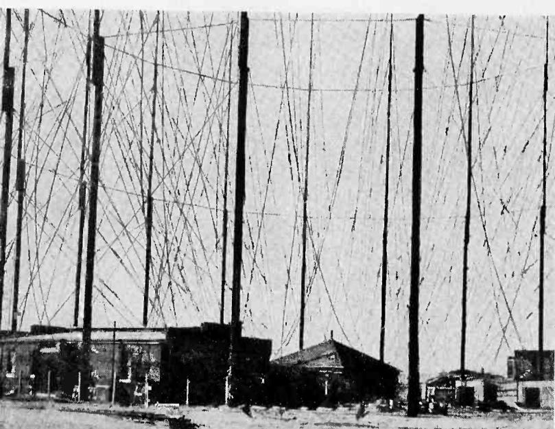
This Marconi radio transmitting station erected at Wellfleet, Mass., in 1902 succeeded in sending signals across the Atlantic.
