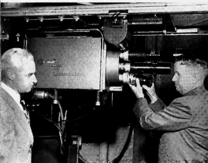
*The first compatible color TV system for medical use was designed by RCA. The TV camera is fitted horizontally and "sees" the subject via a mirror which picks up reflections through an opening in a surgical lamp.*
