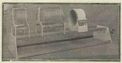
A low-loss tuning unit of skeleton construction exhibited on one of the stands.
