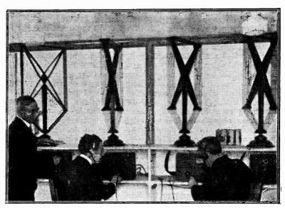
A loud speaker in each apartment and four plug sockets in the walls simplify radio for tenants in one of New York's newest block of flats. A central station on the top floor boasts four radio sets and an operator. Four stations are funed in, and every tenant has the choice of plugging in on one of them. Our photograph shows two of the sets being tuned.
