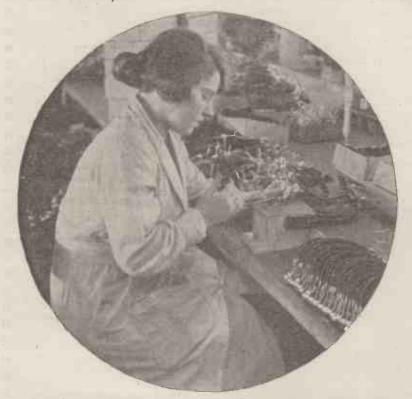
Our photograph shows one of the operations in the manufacture of the B.T.H. headphones. The end of the stirrup is being bent to prevent the slides from coming off.
