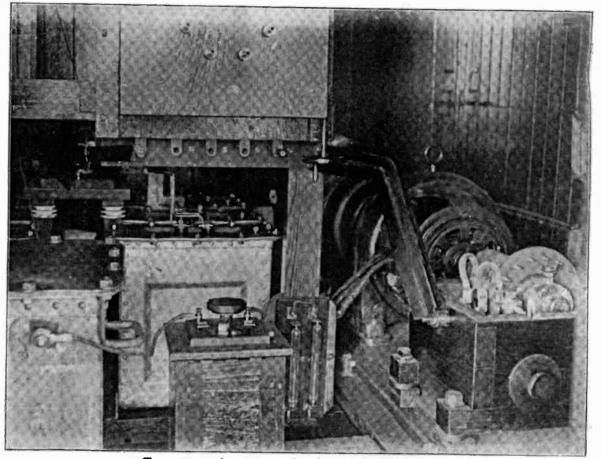
Transmitting Apparatus on board the S.Y. "Mahroussa."
