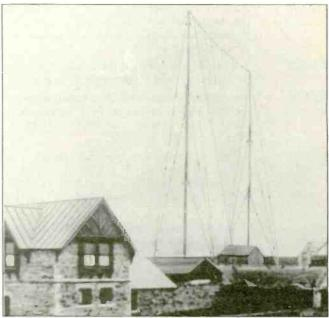
Top left: Inverted cone suspended in a ring of unstayed 200ft masts at Poldhu.
