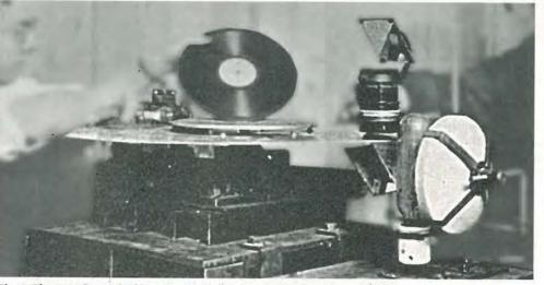
disc underneath the record platter. A light source at the right shines up through the disc via a mirror. This arrangement could also have been used for recording.
