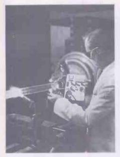
The picture shows the temperature of a silica tube being measured while undergoing a production process. The chopper and temperature sensor form the small unit held in the operator's left hand and pointed at the hot part of the silica tube.
