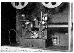
Details of projector mechanism.
