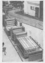
Typical of latest machinery- | Many of the most brilliant | Information on all aspects of | The latest equipment for plastics Prodex sheet plant incorporating a 41" extruder and double shell cooling rolls embodying a built-in heat exchanger.
