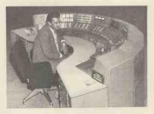
Console of the 34-channel sound mixer manufactured by Pye for the Elstree Studios of Associated Television. In addition to providing mixing facilitles for studio microphones it also provides echo effects and talk-back facilities.
