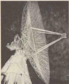
Scanner of the tracking radar inside its I 40-foot radome. Note the sectional construction of the sphere. On the right is the prototype radome housing the tracking radar atop its transmitter-computer building at the R.C.A. experimental establishment at Moorestown, New Jersey. The buildings and radome to be built at Fylingdales, Yorkshire, will be of similar construction.
