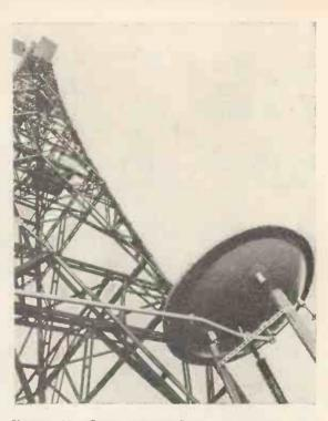
Plane passive reflector on mast reflects to next repeater becm from aerial at ground level.
