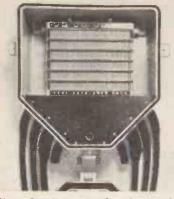
Above: Distribution box for subscribers' lines. Television and/or sound signals can be applied to any subscriber by the insertion of the appropriate resistive or inductive elements which are encapsulated in foamed polyster resin.
