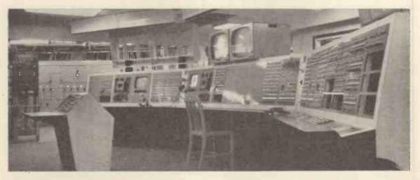
FOCAL POINT of the B.B.C. Television Centre, Wood Lane, London, W.12. All sound and vision signals from the nine studios and the telecine and videotape machines are fed to this Central Apparatus Room for distribution. The first transmission from the centre is on June 29th.
