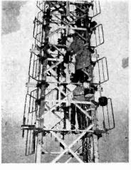
Constructing the Channel 10 aerial installed by Marconi's for the St. Hilary I.T.A. station. It has a gain of 13 giving a vision e.r.p. of 200 kW. The engineers are seen here fitting antiicing shrouds to the dipole supports.
