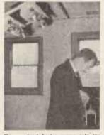
This overhead heater warms only the area within its radiant rays, and so effects a considerable saving of fuel. Its benefits are felt immediately, there is no warming-up period. It is essentially a personal type of heater, having controls within easy reach of the operative. The controls give four variations of heat and "Off." At maximum heat the unit consumes 1 kW.
