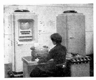
Decca Radar digital computer using magnetic-core circuits.
