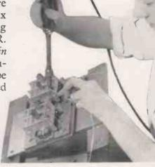
At the Plessey Company Limited's Works, Ilford, where Ersin Multicore Solder is used for bridging the gap between the stator vanes and terminals of variable condensers.
