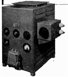
This is the Rediffusion R.H.2, delivering more than 250 watts of radio frequency power. Only 18 x 15 x 12 inches, it is very simple to instal and control. The matching unit shown on the bracket may instead be coupled to the set through a 6-ft. screened cable.
