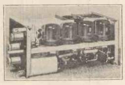
GERMAN CARRADIO. The new all-metal valves have been used extensively in the new car-radio receivers which were to be seen at the Berlin Motor Show. There is no waste space in the 6-valve Körting receiver, shown here.
