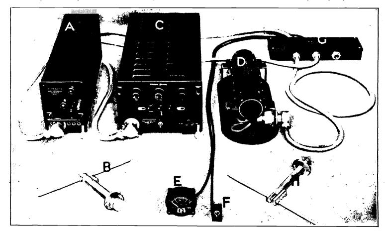
The various units of the altimeter equipment. A, receiver; B, transmitter dipole (length is about rin.); C, power supply unit, including HT generator; D, UHF oscillator; E, indicating meter, calibrated in hundreds and thousands of feet; F, range switch (hundreds to thousands of feet);
