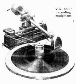
With the Simplat recording blanks which have a comparatively soft surface the drag imposed during cutting is not heavy, and this fact greatly facilitates the use of existing gramophone motors.
