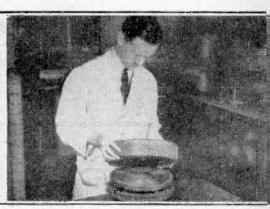
The finished record is next held up to the light to see how loud it has been recorded, and when satisfied with the finished product bronze powder is whisked above. The purpose of the bronze powder is to provide metallic contact for electro-plating. The wax is next mounted in an ebonite shell and, in this containe form of ridges instead of grooves. This master negative is too valuable to be used f
