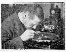
opphire point and the wax is then examined through a magnifying glass to see that everything is in order. So as to ensure smooth running a gravity motor incer keeps an eye on it to see that the fine spiral cut by the sapphire point is being drawn off correctly by suction, and when the record is completed the eer examines the grooves under his magnifying glass.
