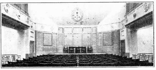
Fig. 6.—General view of the stage in the assembly hall showing sloping ceiling in front of loud speakers.
