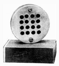
The miniature microphone compared with a box of matches.
