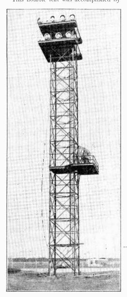
An engineer of the Western Electric Company shows how the super-power scund projector may be trained upon a distant "target" so that voice or music may be delivered to that point without wasting acoustic energy over a large area
