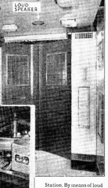
speakers passengers are warned to '' Stand Clear of the Doors '' before these are automatically operated. The system employs an amplifier and a photo cell fed from a controlled sound track on a continuous belt of film, illuminated by a 12-yolt lamp. A by a 12-volt lamp. A spare lamp automatic-ally comes into opera-tion should the original one burn out.
