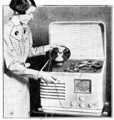
THE DUO-TRAC SOUND PROJECTOR, which is being shown and demonstrated at the British Industries Fair at Olympia, has the sound recorded on a film which gives 30 minutes' playing time with a spool of standard size. The apparatus shown above is a table model and embodies an all-wave radio chassis.
