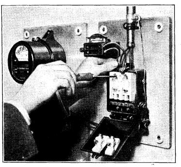
Reproduced from "Interference Suppression" by courlesy of Belling & Lee, Ltd Fitting a condenser suppressor to the main fuse-box.
