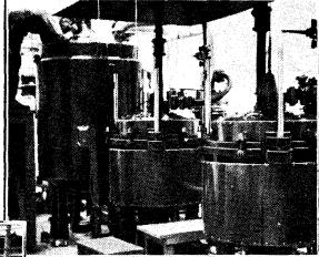
A certain element of secrecy surrounds the methods employed for producing electrolytic condensers, and the rolled paper dielectric condensers are also turned out by machines of a special design. The latter type are impregnated in vacuum ovens and slowly cooled off to prevent crystallisation of the wax and the absorption of water.
