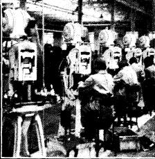
Here nuts, screws and spindles are turned out by the automatic lathes, while coil cans, laminations, switch contacts, etc., are produced by the automatic toggle presses. A huge automatic cadmiumplating plant has just been installed in which a chain conveyor takes the chassis parts through cleaning and washing baths, and, after passing at a regulated speed through the plating vat, finally dries the products in a hot-air oven at the far end.
