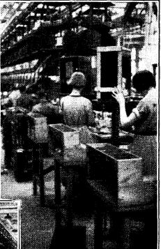
(Above) Assembling chassis and cabinets. Note the pneumatic hoists.
