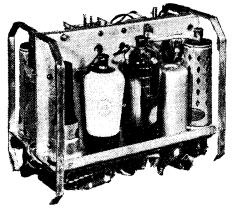
Chassis of Marconiphone car radio receiver.
