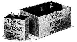
T.M.C.-Hydra condensers for use in highvoltage circuits.
