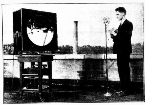
Parabolic mirrors are used for ULTRA-SHORT WAVES AND THE MICROPHONE. "beamcasting" at the Chicago Century of Progress Exposition. This is the apparatus under test. Its sponsors guarantee that, unless the beam is intercepted. complete privacy is secured.
