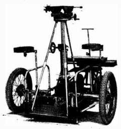
A tracking truck designed to transport the microphone boom noiselessly from point to point in the studio.
