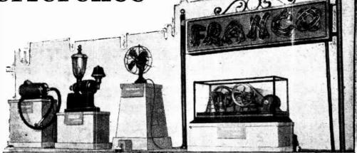
Types of local interference. The electric sweeper, coffee roaster, fan and flashing sign.
