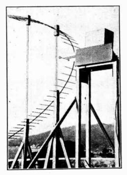
A receiver for the quasi-optical wavelength of 50 centimetres recently used by Marchese Marconi.
