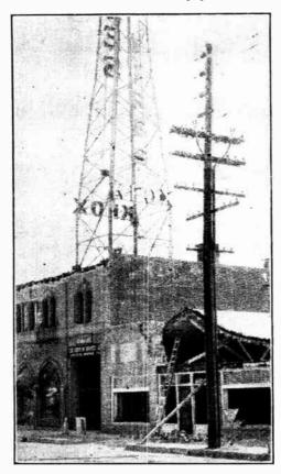
A REAL BREAKDOWN. B.B.C. are spared such calamities as befell KFOX Long Beach in the heart of the Californian earthquake zone. The photograph indicates that the mast and near-by telegraph poles withstood the shocks better than the building.
