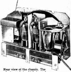
adaptor socket, which is used only when batteries are employed, can be seen on the extreme right,
