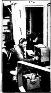
WIRELESS FOR NAVAL SURVEY. On the left is H.M.S. Challenger, which has just left Portsmouth to carry out survey work, with the aid of wireless, off the coasts of Labrador. Note the D.F. aerial on the bridge. Above: Sailors examining transportable sets.
