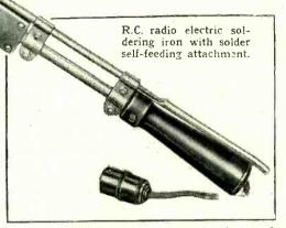
The copper bit is of generous size, and quite suitable for all normal requirements, and models can be obtained for use on supply mains of from 100 to 250 volts, either A.C. or D.C. For an additional sum of 3s. a self-feeding attachment to hold a stick of solder not exceeding sin. in diameter can be obtained.
