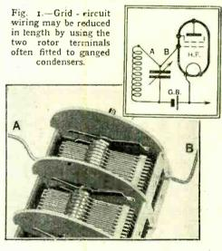
valve on one side of the condenser and the coil on the other, and it is a good plan in such cases to make use of both connection points in the manner suggested in Fig. 1, where the wirds in question, which bear corresponding lettering, are shown both diagrammatically and pictorially.
