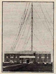
MOORSIDE EDGE. A photograph taken last week showing the newly completed station building for the Northern Regional transmitter. The design is identical with that of Brookmans Park. The masts are 500 feet high.
