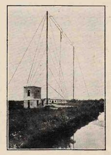
"EIAR RADIO MILANO." — The picturesquely situated station which works in close association with Radio Turin and is like that station in having a lady announcer. It can readily be heard in England, working on a wavelength of 501 metres with an aerial output of 8 kW.
