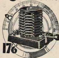
"HIS is a Wave Trap as well as Ta Tuner. It gives sharp tuning and eliminates interference. Its special winding, designed to give loose aperiodic coupling, explains the life and definition which it gives to the tuning of any circuit in which it is incorporated.
