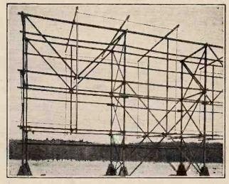
One end of a short-wave receiving aerial erected by the Bell.
