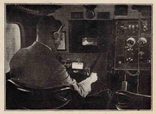
The Fultograph receiver in use in a Lutthansa aeroplane. To prevent spilling, a sponge soaked in potassium iodide solution was employed in the experiments. On the right is the Telefunken transmifter and receiver.
