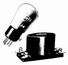
The Mullard high magnification factor pentode output valve and the Permacore transformer with nickel and silver windings.
