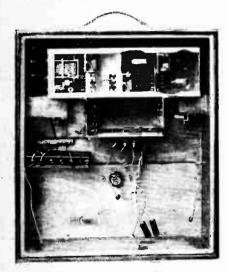
View of the interior of the new McMichae portable set. Elaborate screening is arranged for the two screened-grid valves.
