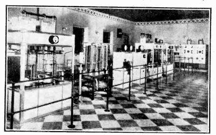
BROADCASTING FROM ITALY. Maximum efficiency is suggested by the spick and span appearance of the Milan transmitter, seen in the photograph. Built by the Marconi Company for the Unione Radiofonica Italiana, the transmitter yields an aerial power of 7 kilowatts. The main panels use water-cooled valves, the water being sprayed into tanks mounted on the top of the frames.
