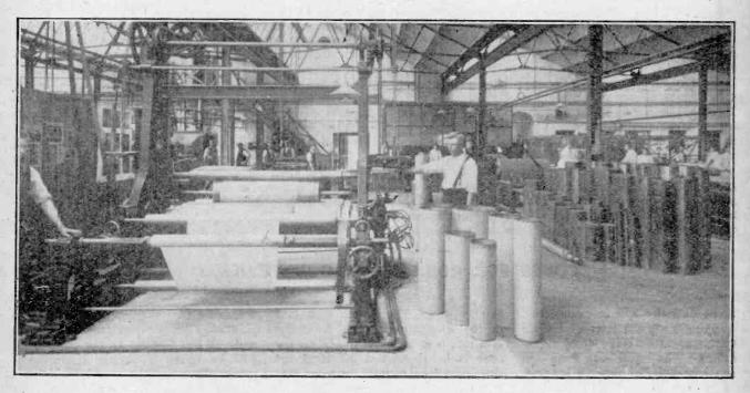
Fig. 4.--A tube-winding machine. The bakelised paper is slowly wound round mandrels against which electrically-heated rollers apply a heavy pressure.
