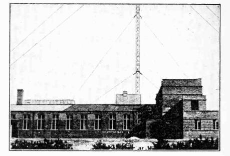
WESTERN EUROPE'S BIGGEST STATION.—Part of the station building and aerial at Zeesen, near Konigswusterhausen. The new station, which uses a power of 40 kilo-watts on a wavelength of 1,250 metres, will shortly supersede the original station at Konigswusterhausen.
