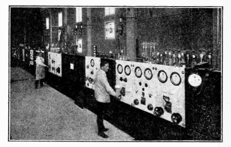
FAMOUS GERMAN COMMERCIAL STATION,—A photograph taken in No. 3 Trans-mitter House at the Koenigswusterhausen telegraph wireless station. The 10-kilowatt valve transmitter working on 2,865 metres is on the extreme right; in the centre is a reserve 2-kilowatt transmitter and on the left the 2-kilowatt "Deutschland Sender."
