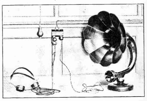
A typical reception point. Note specially the volume control on the plug attached to the telephone.
