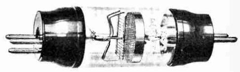
Fig. 4.—The new screened valve in the Marconi and Osram series type.
