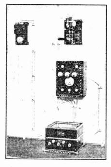
AUTOMATIC S.O.S. DEVICE. A new instrument designed by the Marconi Company which gives audible warning hymeans of a bell when an S.O.S. message is received. The employment of this device, which is provided for in the Merchant Shipping (Wireless Telegraphy) Rules just issued by the Board of Trade, dispenses with the necessity for maintaining continuous wireless watch on board ship.
