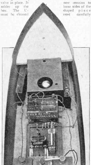
A general view of the screened radio receiver, with the relay panel in the foreground.
