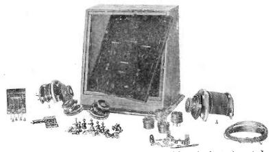
Complete set of finished parts for building a high grade three-valve set, by Messrs. L. McMichael, Ltd.
