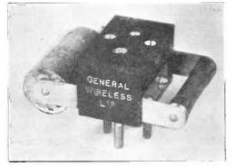
[General Wireless, Ltd. Fig. 1. Attachment for providing grid potential and resistance across transformer winding.
