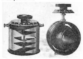
Maxone variable condenser with specially shaped plates and variometer by Messrs. J. Macdonald & Co.
