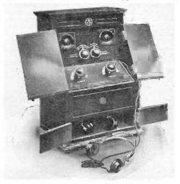
B.T.H. 2-value receiver showing receptacle for head telephones.
