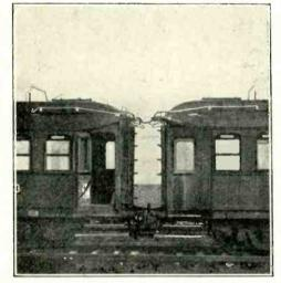
The brackets on the extreme left and right support the aerial wires. The lead between the compartments is the connecting cable.
