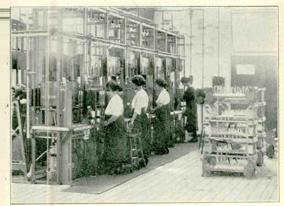
The value pumping plant. Each operator deals with a batch of about 20 values. The filaments are run at a high temperature and a high voltage is applied to the anodes. The filament current of each value is adjustable by the operator, and during the pum ing the current is varied according to the degree of vacuum.
