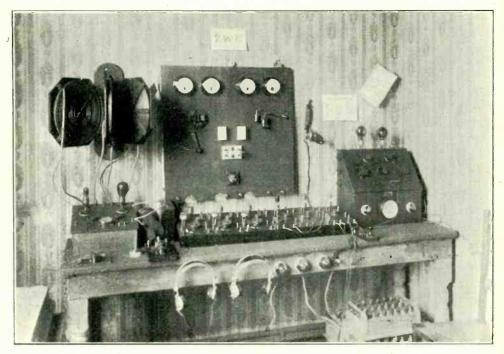
The experimental transmitting and receiving equipment at 2 WK, the station of Mr. G. R. Lewis.
