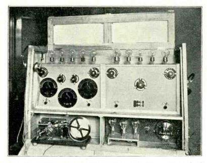
The apparatus for the elimination of atmospherics during the reception of signals on long wavelengths.
