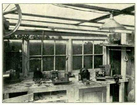
Another view of the workshop. It will be noticed that both gas and electric light are available. The provision of ample cupboard space and racks is essential where the workshop dimensions are limited.
