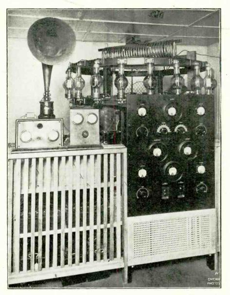
The layout of the transmitting gear at the **Chicago** Broadcasting Station, shown above, is of interest as it differs very much from the arrangement employed at the British broadcasting stations. Fower is derived from a 10 kW. generator at 4,000 v.
